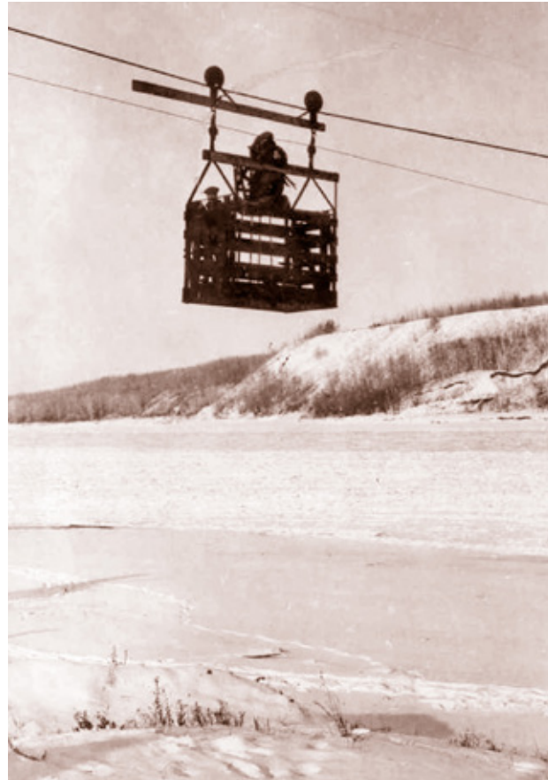
The cable cage that carried passengers across the Athabasca River in the spring and fall from 1934 to 1952. Athabasca Archives, 00870.
